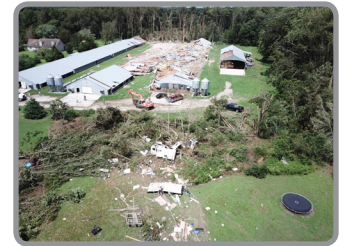
Tornado damage in Stockton, MD. Credit: NWS AKQ
