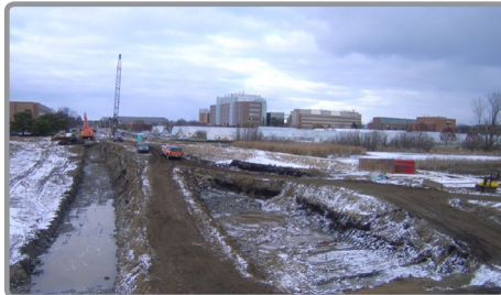
Wintertime construction in Michigan. Image: MSU IPF (via Flickr CC)
