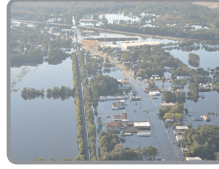
Flooding in Lumberton, NC. Credit: SCEMD and Civil Air Patrol
