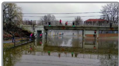
Flooded underpass on April 28 Fredericton, N.B. Credit: Rick Fleetwood.
