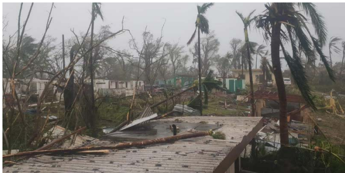
Severe devastation on Saipan from Super Typhoon Yutu. Photo from Business Insider .
