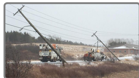
Ice and strong winds snapped power poles in Saint John, NB, on February 27. Credit: Roger Cosman CBC New Brunswick.
