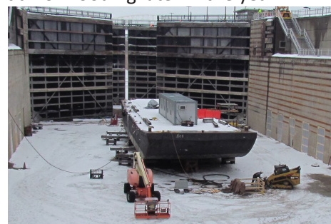
Repair at the Soo Locks (credit: USACE).
