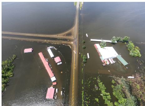
Flooding on Illinois Highway 3 in late June in southern Illinois. (Illinois DOT)
