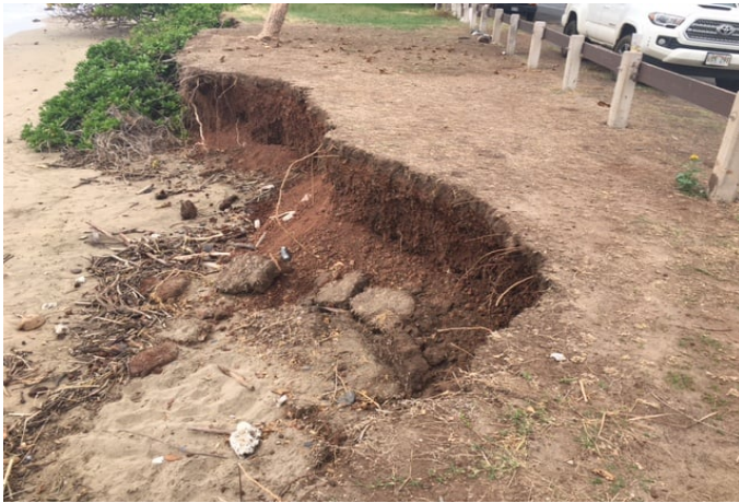
Coastal erosion leading to park closures in Jan.-Feb. at Puamana Beach Park, Maui. Photo credit: Maui Co.
