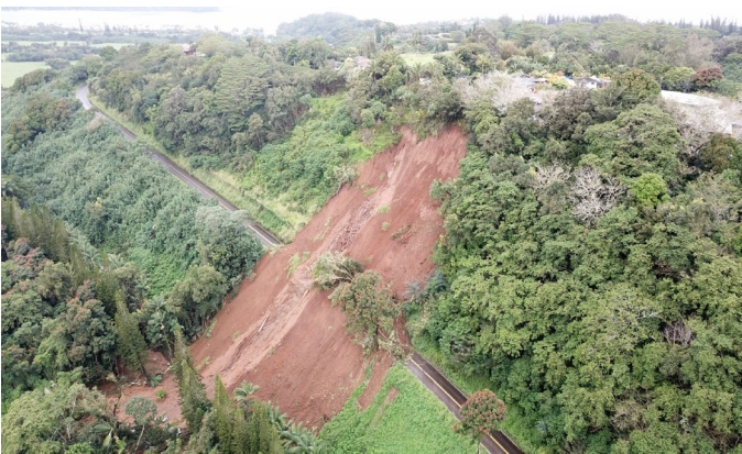
Hanalei Hill landslide on Kuhio Highway (Kauai) during the March 2021 heavy rainfall and flooding events. Photo credit: Hawaii Department of Transportation.
