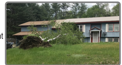
Tornado damage in Sullivan County, NH. Photo credit: NWS Gray
