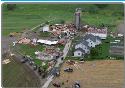
Damage from an EF-1 tornado in Lancaster County, PA, on May 27. Photo credit: NWS State College
