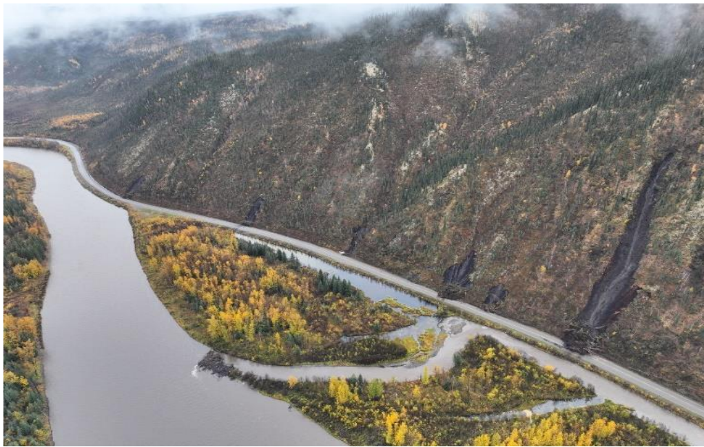
Landslides on North Klondike Highway Photo credit: Yukon Government
