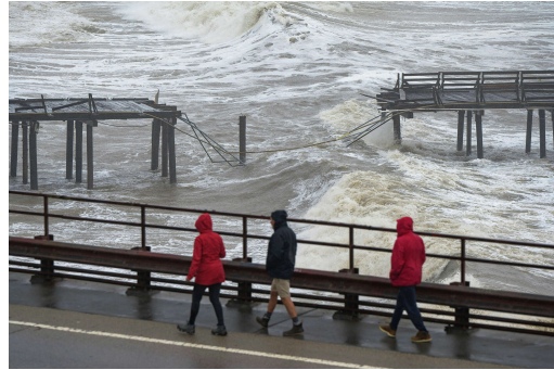
Image: Damaged Capitola, CA Wharf on 5 January, 2023. Credit: Nic Coury/AP
