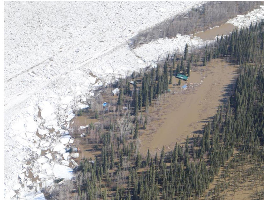
Buildings flooded up to the roof at Forty Mile Photo credit: Government of Yukon
