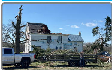
Tornado damage in Sussex County, DE, in April 2023. Credit: NWS PHI
