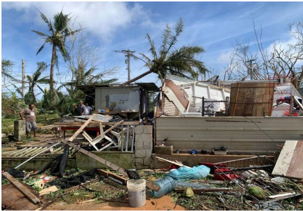
Wind and flood damage to home in Yigo, Guam following the passing of Typhoon Mawar. Image credit: Red Cross, Guam.
