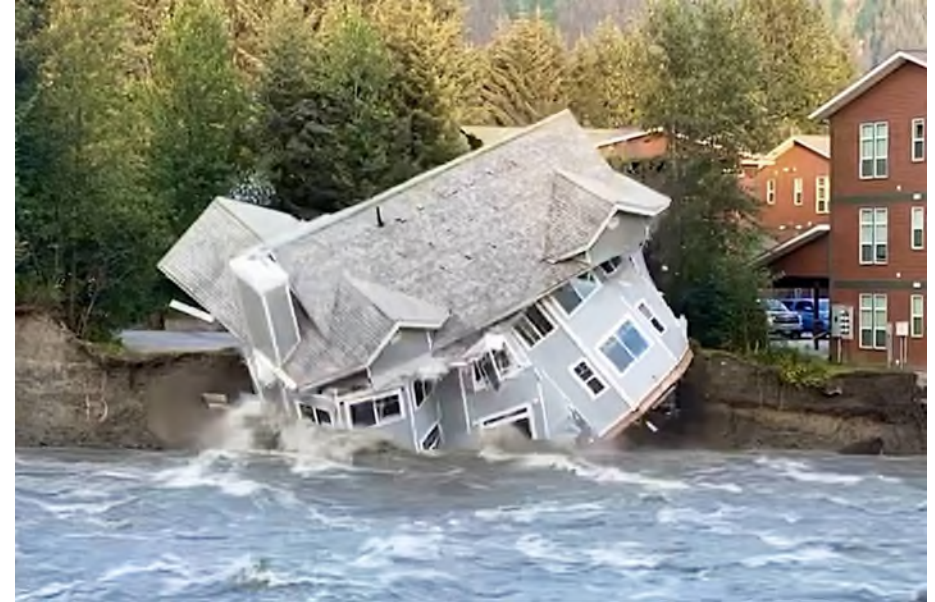
A Juneau house collapses into the Mendenhall River after erosion undercuts bank. Photo credit: Sam Nolan
