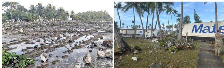
Flooded runway and debris at the Woja Island Airport, Ailinglaplap Atoll, RMI (above left). Storm surge damage to infrastructure in Roi-Namur, Kwajalein, RMI (above right). Source: Marshall Islands Journal; U.S. Army.
