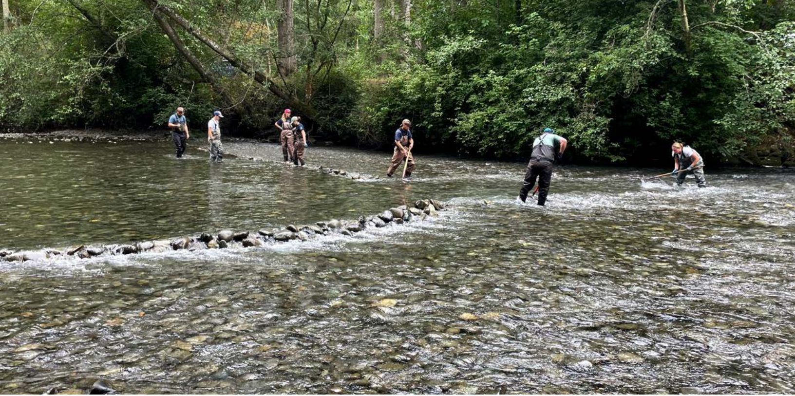
Figure 24: Crews modify a low flow barrier riffle on the Dungeness River to assist fish passage during drought (credit: Chandra Johnson, Jamestown S’Klallam Tribe).
