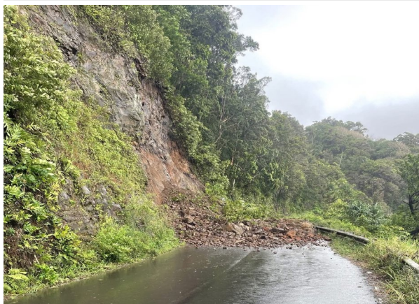
Landslide in association with heavy rains and saturated soils along Hana Highway between Kaumahina State Wayside Park and Kanae Peninsula in Maui (2/9/26).
