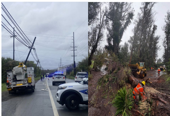
Wind damage including downed power lines and trees in Maui (2/9/26).
