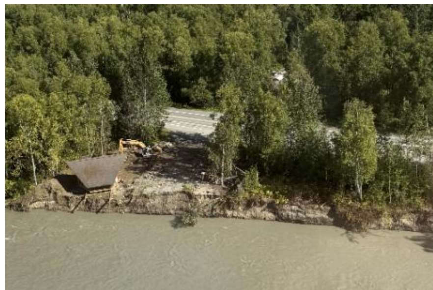
Photo showing severe riverbank erosion and damaged structures. Photo credit: Katie Writer ( https://cubflights.com/ )
